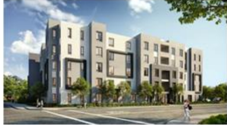
66 Units of MFH with 17 set aside units.
